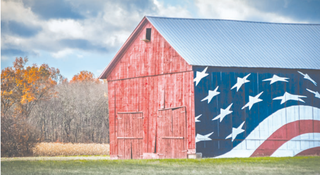
A newly painted tobacco barn in West Suffield as seen on Mountain Road.
